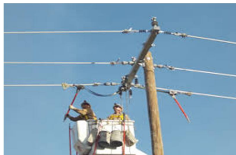
Fig.2 shows hot stick method using insulated sticks
