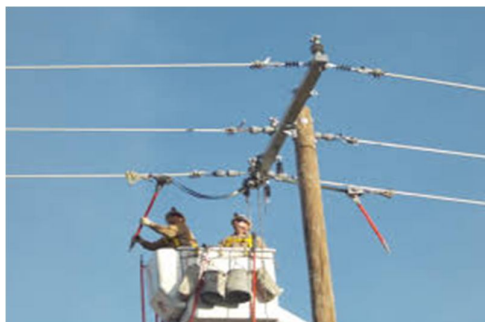
Fig.2 shows hot stick method using insulated sticks
