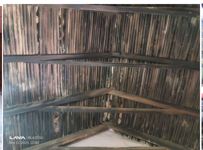
Bamboo roofing at the entrance porch
