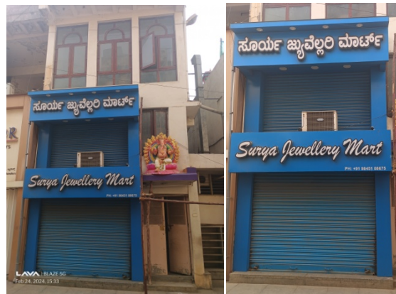
AcP cladding façade with metal rolling shutter
