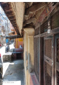
Bamboo roofing at the entrance porch
