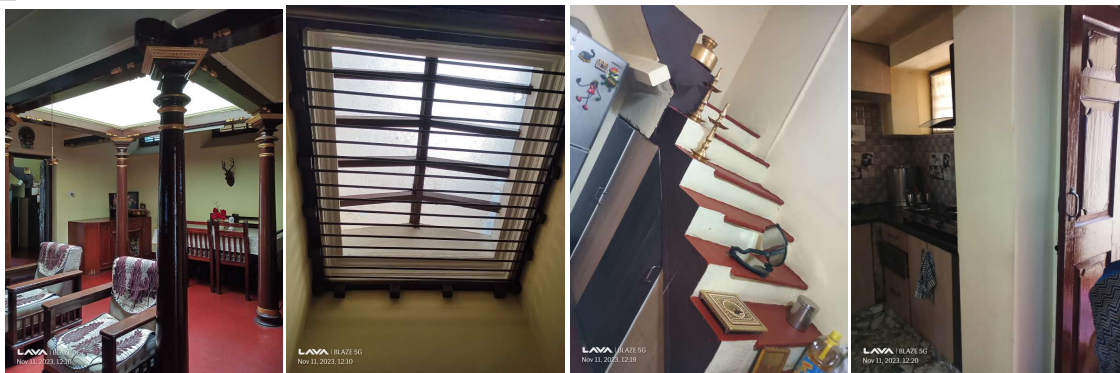
Courtyard which is now used as skylight
