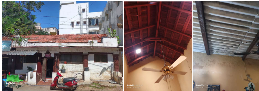
Front facade Converted courtyard into living room Use of slate roofing sheets
