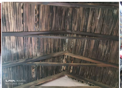
Bamboo roofing at the entrance porch
