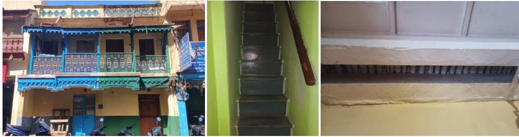
Front facade 600 mm width staircase Structural roofing system made with bamboo
