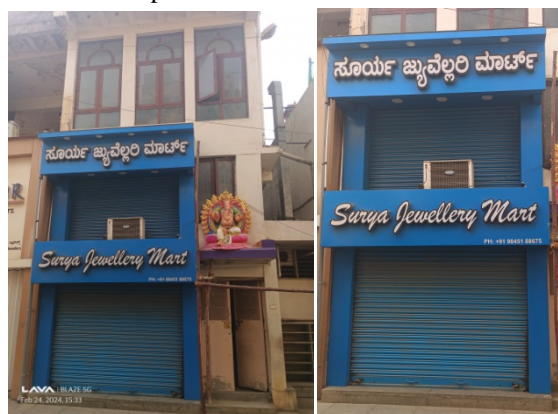
Acp cladding façade with metal rolling shutter
