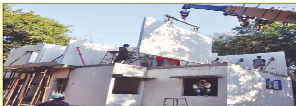
Figure 2 Construction of GFRG panel house
