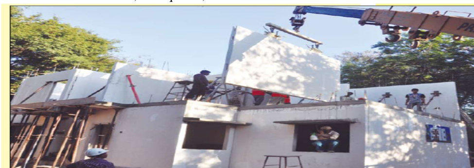
Figure 2 Construction of GFRG panel house
