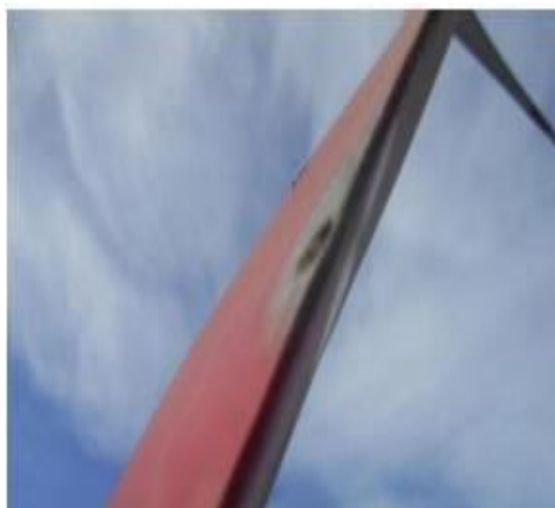
Figure 5: Lighting Damage.
