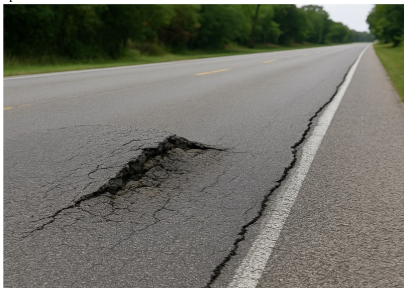
Figure 1: Pavement uplift and longitudinal crack caused by expansive soil
