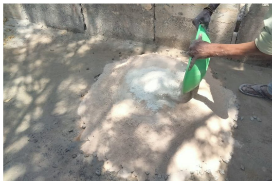
Figure 4.1: Dry mixing of aggregates and binders
