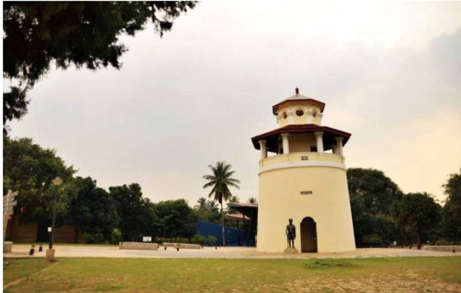
Fig 4: The reused “watchtower”
