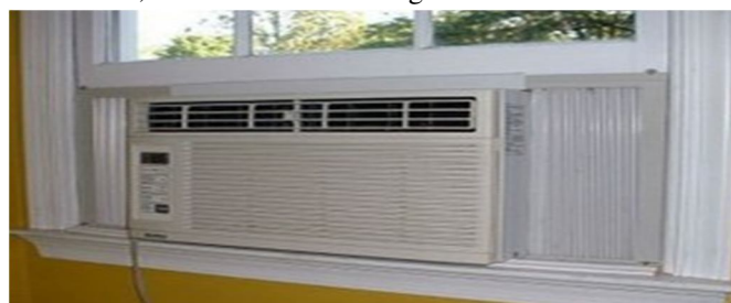
Fig a) Window unit and packaged terminal
