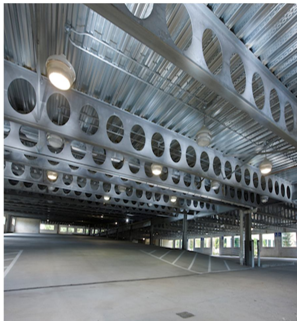
Fig. 2: Typical Steel Beams with Openings in the Web
