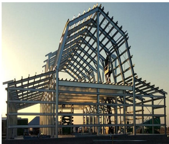
Fig. 1: Industrial Steel Structure
