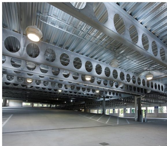
Fig. 2: Typical Steel Beams with Openings in the Web
