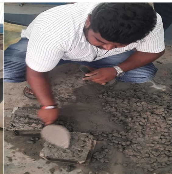
Fig 4: pouring of concrete
