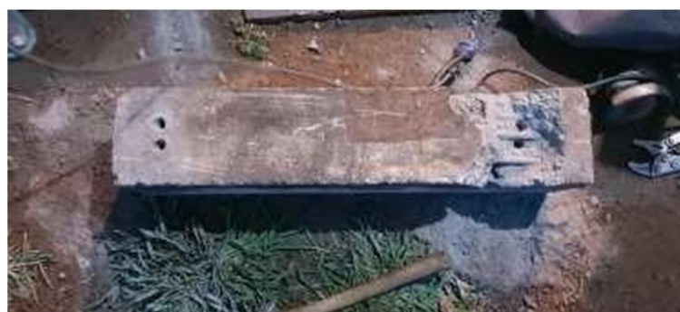
Figure 8.8: Drill pattern of holes for stitching method
