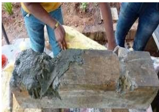
Figure 8.5: Sealing pot holes and spalled portions with repair mortar
