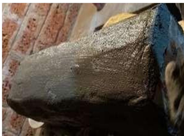
Figure 8.11: After rehabilitation by Meshing + Stitching method
