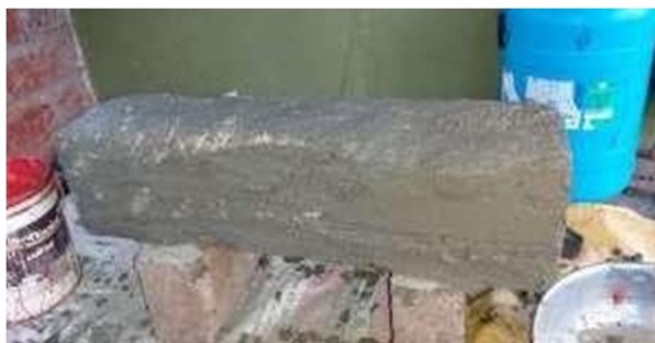
Figure 8.6: Application of repair mortar over three sides of beam
