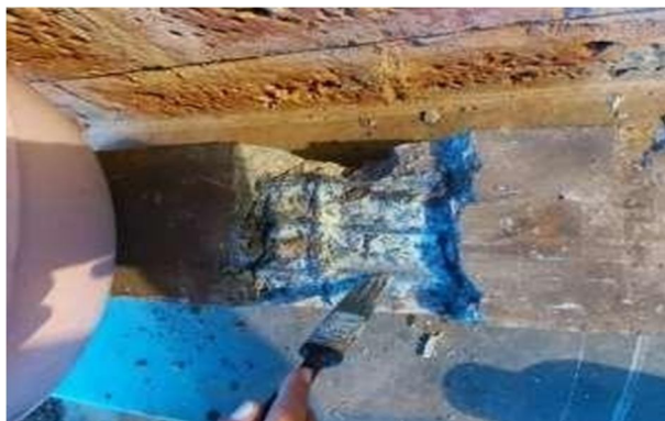
Figure 8.4: Application of Rust remover on the reinforcement
