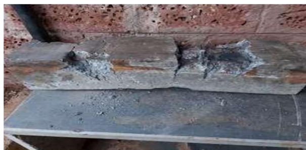
Figure 8.3: Removal of damaged concrete
