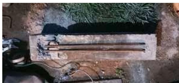
Figure 8.9: Placing of U shape bars into the beam
