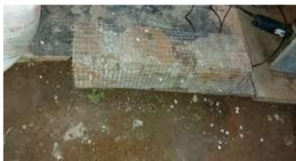
Figure 8.7: Placing of stainless steel mesh on the three sides of beam
