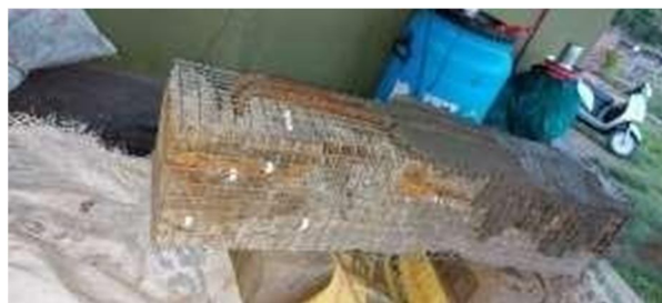
Figure 8.10: Application of repair mortar
