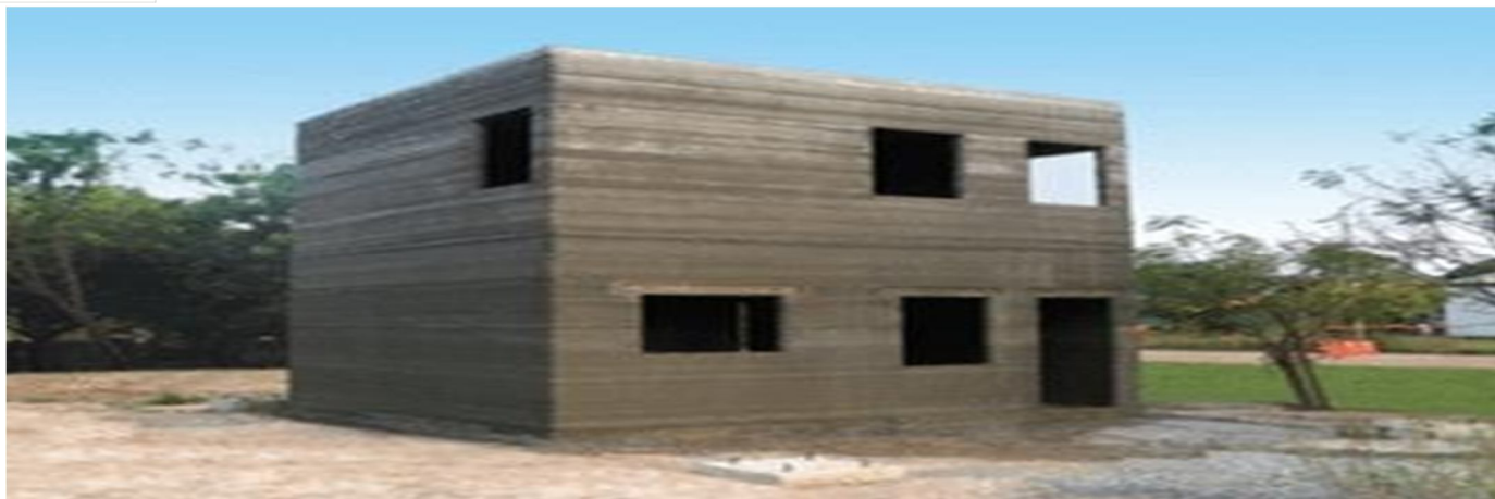
FIG. 10. Image of 3D Printed Two-Storey Building.
