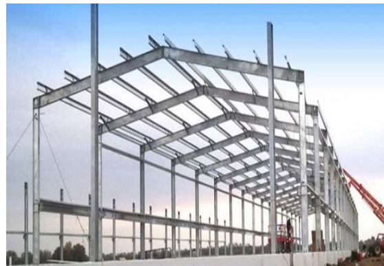
Fig. 1 Cold-formed steel structure
