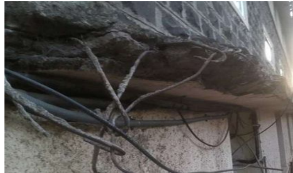
Figure 8: Exposed reinforcement
