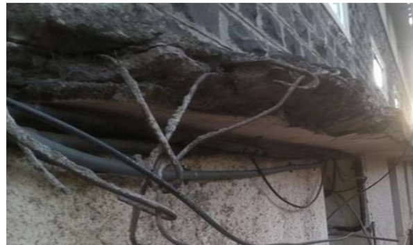
Figure 8: Exposed reinforcement
