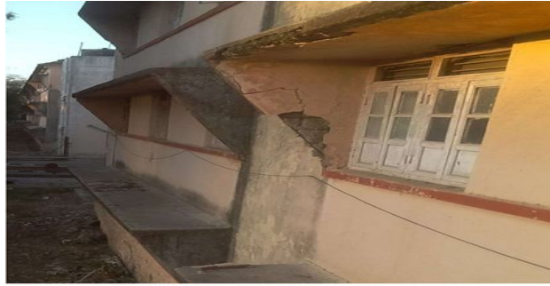
Figure 7: Cracks in chajja
