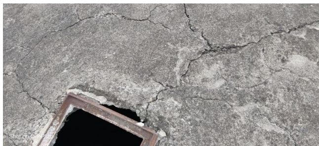
Figure 4: Cracks in slab of ESR
