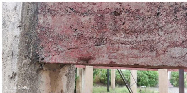
Figure 6 : Cracks in bracing
