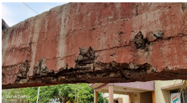
Figure 5 : Exposed and reinforcement at bottom of bracing
