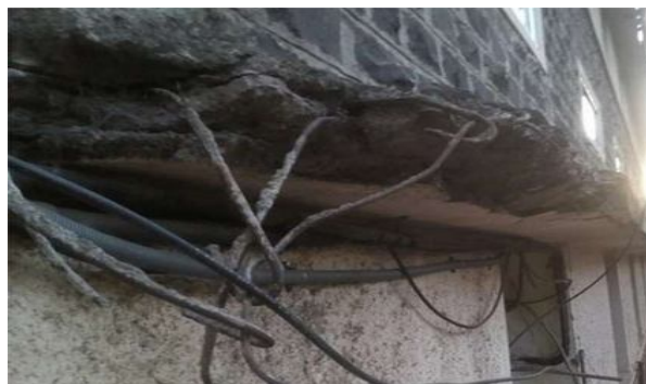
Figure 8: Exposed reinforcement
