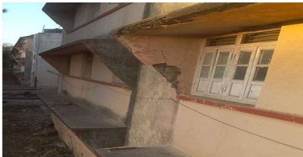
Figure 7: Cracks in chajja
