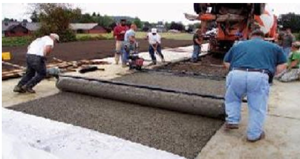
Fig 6 Compaction of pervious concrete with a steel roller.(R. Banka)
