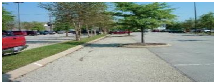
Fig.2 pervious concrete pavements for parking lots
