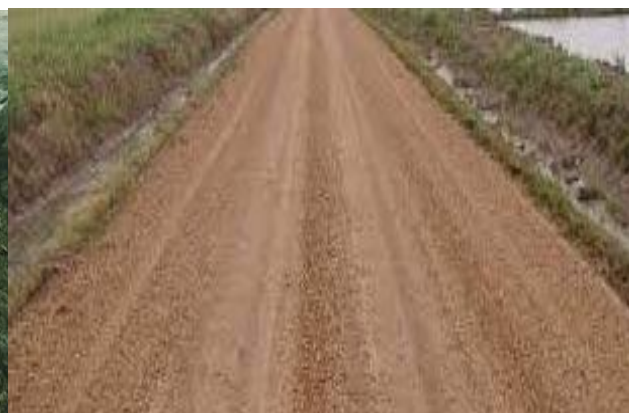
Figure 9 Formation of ruts in reinforced section
