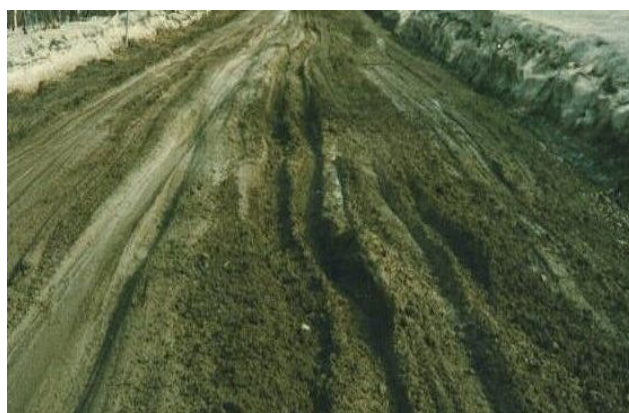
Figure 8 Formation of ruts in un reinforced section
