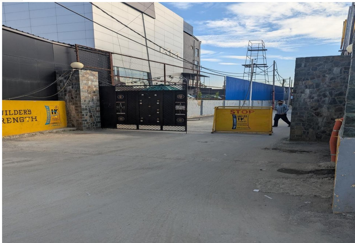
Fig. 4.2. H.K Cement Plant
