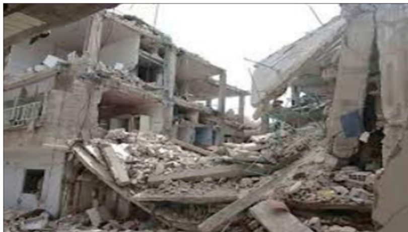
Figure 1.1: School Building Collapse in Lagos, Nigeria 2019
