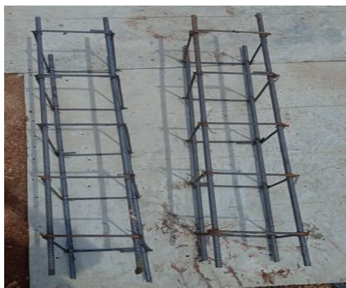
Fig. 8 Reinforcement Work of Column
