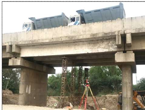
Fig 1: - Bridge Load Testing
