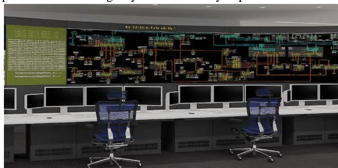
Figure 8: Medical Emergency Unit Control
