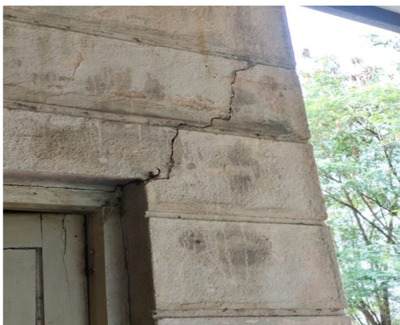
Fig. Diagonal crack formation
