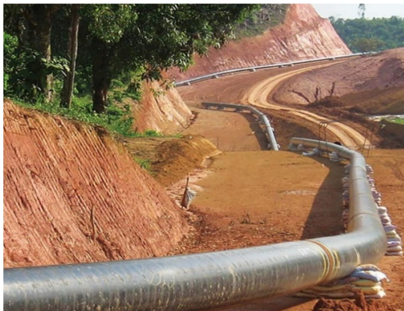
Fig. 2 – Bends in slurry pipelines.
