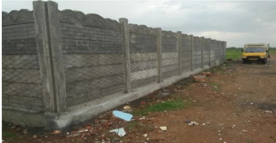
Fig. 7 Precast Compound Walls
