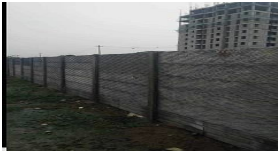
Fig. 8 Precast Compound Walls
