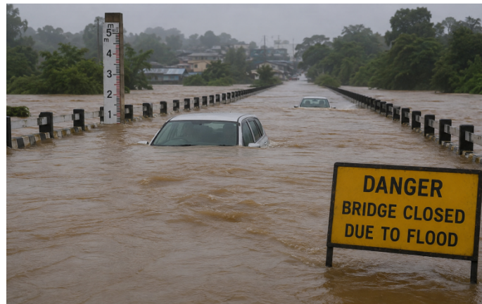
Fig 2. Flooded Bridge During Heavy Rainfall
