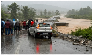
Fig 3: Unsafe Vehicle Movement / Blocked Bridge Due to Flood
