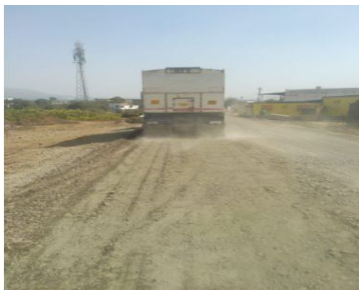
Fig. 1 Cement Spreading
