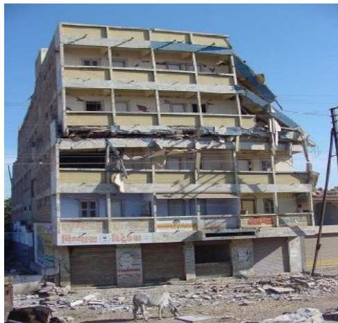
Soft Storey Failure of Building
