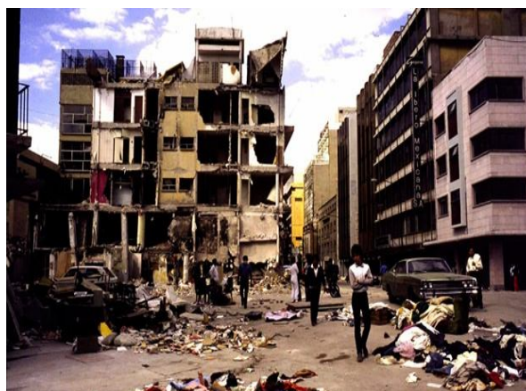
Collapsed buildings with mass irregularity
