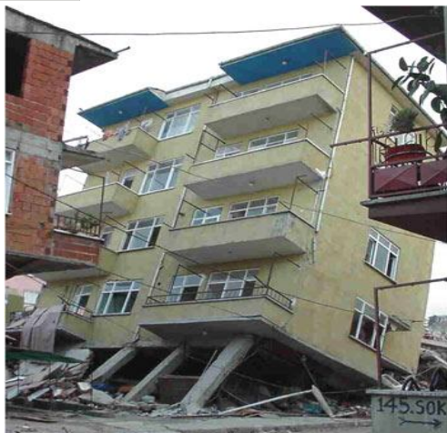
Soft Storey Failure of Building
