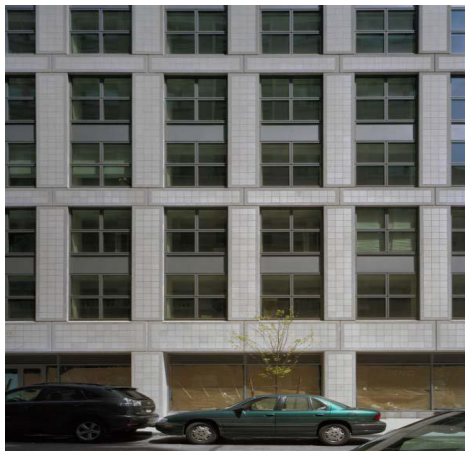
Building with floating column
