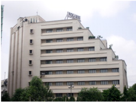
Fig-1 Vertical geometric irregularity in stepped building frames Fig-2 Vertical structural irregularity
