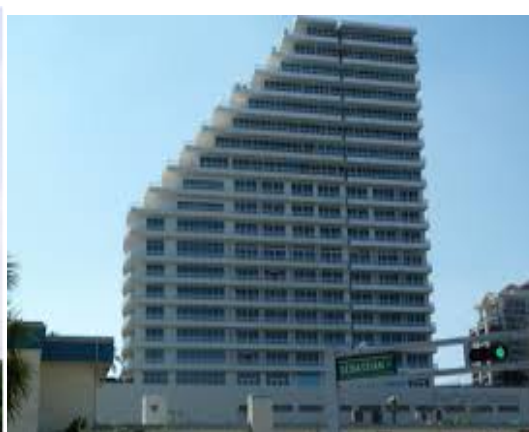
Fig-1 Vertical geometric irregularity in stepped building frames Fig-2 Vertical structural irregularity
