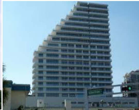
Fig-1 Vertical geometric irregularity in stepped building frames Fig-2 Vertical structural irregularity
