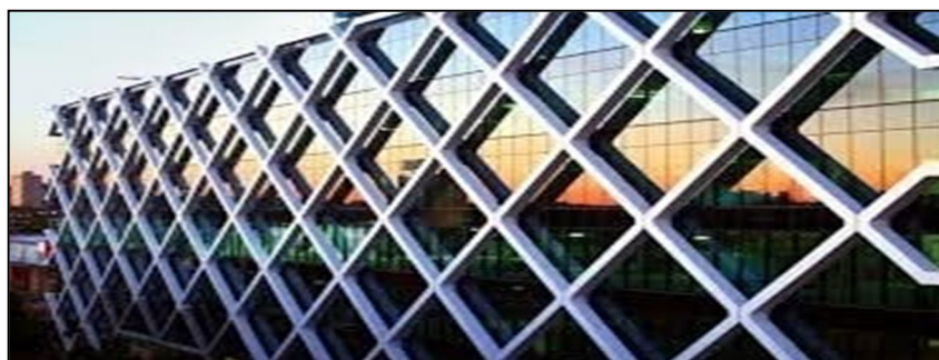
Figure 1: Steel Diagrid Structural Systems
