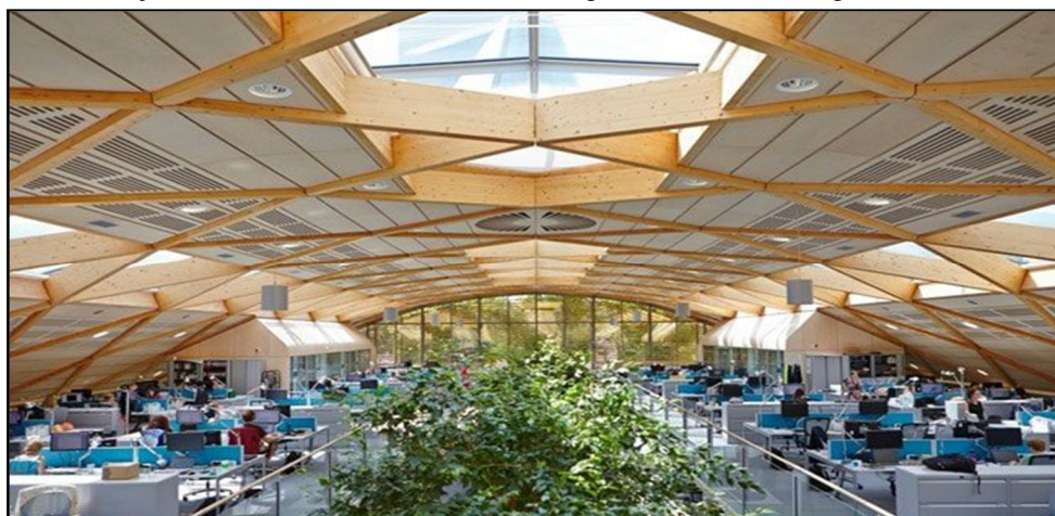
Figure 3: Timber Diagrid Structural System
