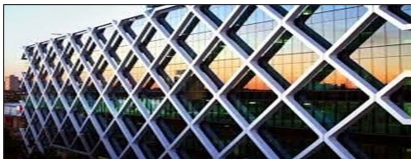
Figure 1: Steel Diagrid Structural Systems
