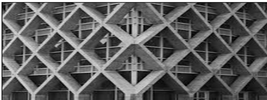
Figure 2: Concrete Diagrid Structural System
