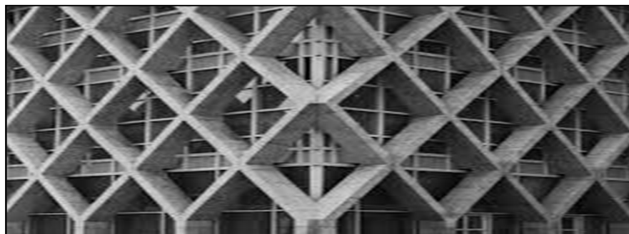
Figure 2: Concrete Diagrid Structural System
