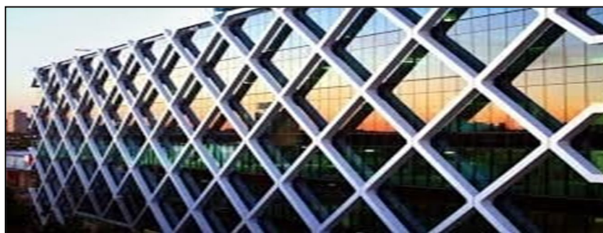
Figure 1: Steel Diagrid Structural Systems
