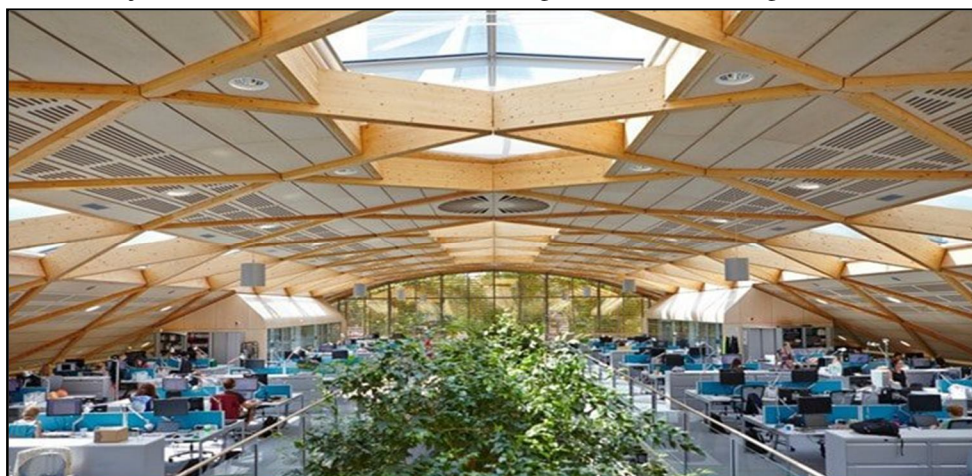
Figure 3: Timber Diagrid Structural System
