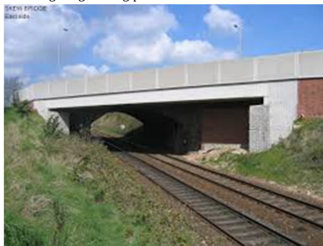
Figure 1. RCC skew bridge
