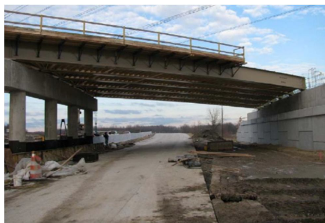
Figure 2. Steel Skew Bridge
