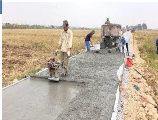
Fig.3.2 laying cement concrete road
