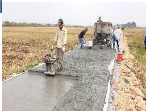
Fig.3.2 layingcementconcrete road
