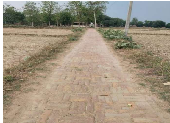
FIG 5.2 COMPACTION AND FINISHING
