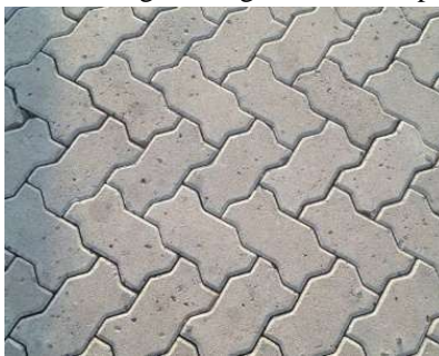
FIG1.1: CONCRETE PAVER BLOCK (200*160*80)mm
