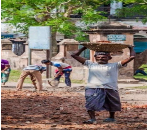
FIG4.2 LAYING OF SURFACING MATERIAL
