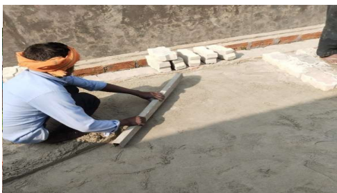
FIG4.1 LAYING OF SURFACING MATERIAL
