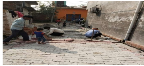
FIG 5.1 COMPACTION AND FINISHING
