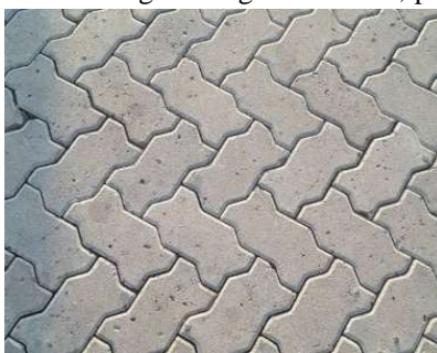
FIG1.1: CONCRETE PAVER BLOCK (200*160*80)mm
