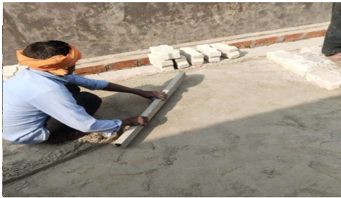
FIG4.1 LAYING OF SURFACING MATERIAL
