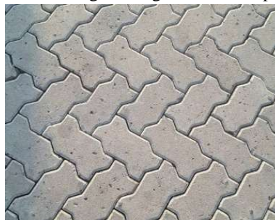
FIG1.1: CONCRETE PAVER BLOCK (200*160*80)mm
