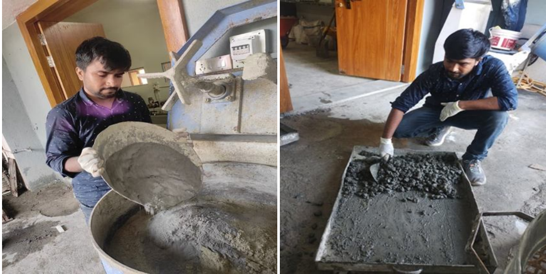
Figure 1: Concrete Mixing and Batching
