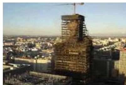
Fig. 1 The Windsor Tower’s fire, Madrid (2005): a) full developed fire, b) post-fire damaged structure.
