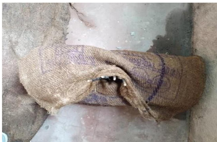
Fig.No.3.17) Curing of Beam
