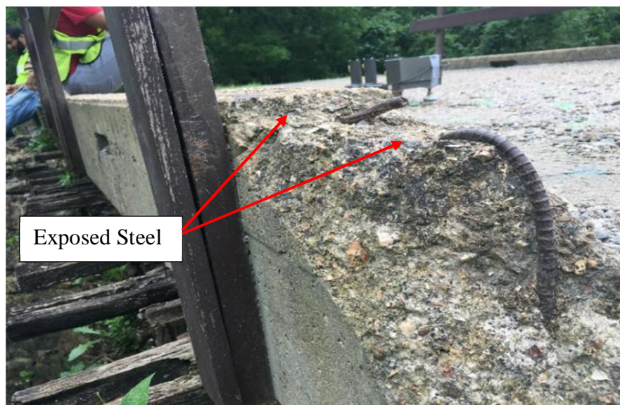
Figure 4. Visual evidence shows the exposed reinforcement steel bar. (In the picture is a corroded steel bars on the girder.)
