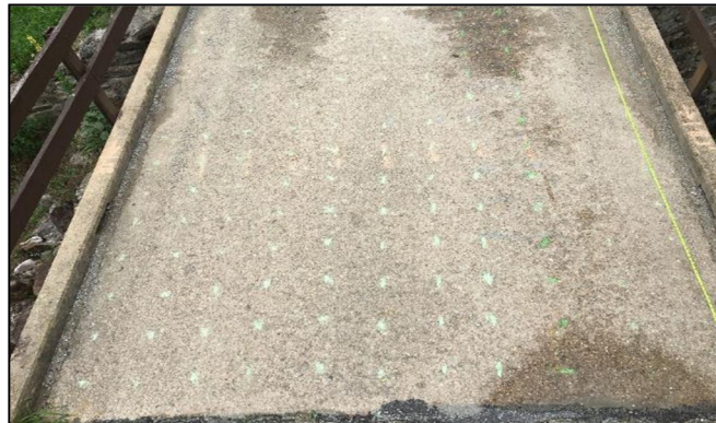
Figure 2. Visual evidence of loss of concrete surface.
