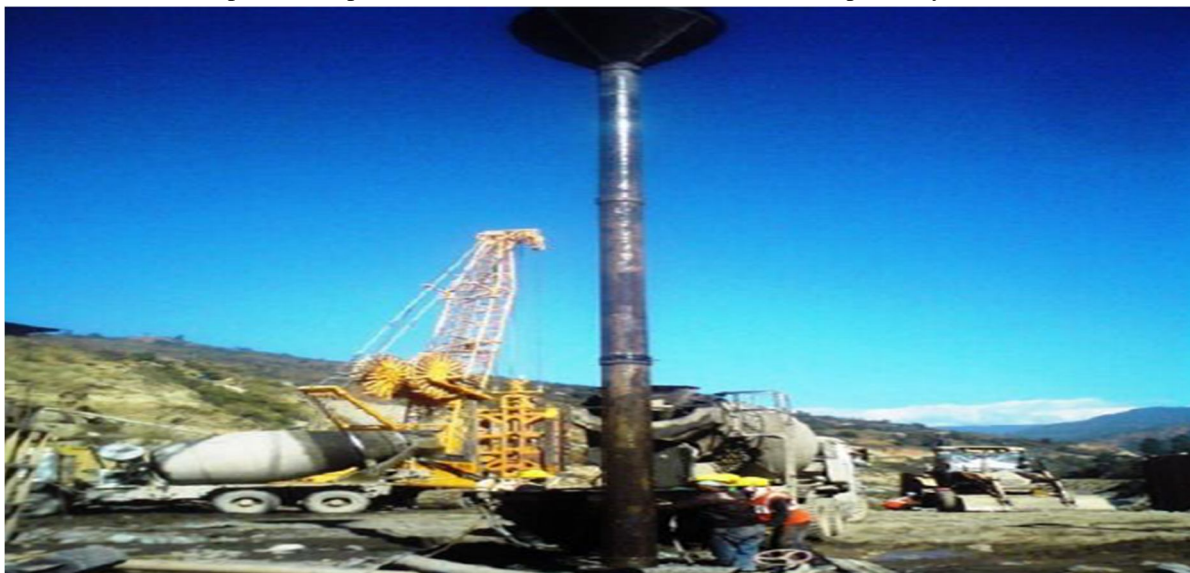
Fig 11.1. Concreting of Panels via Tremie
