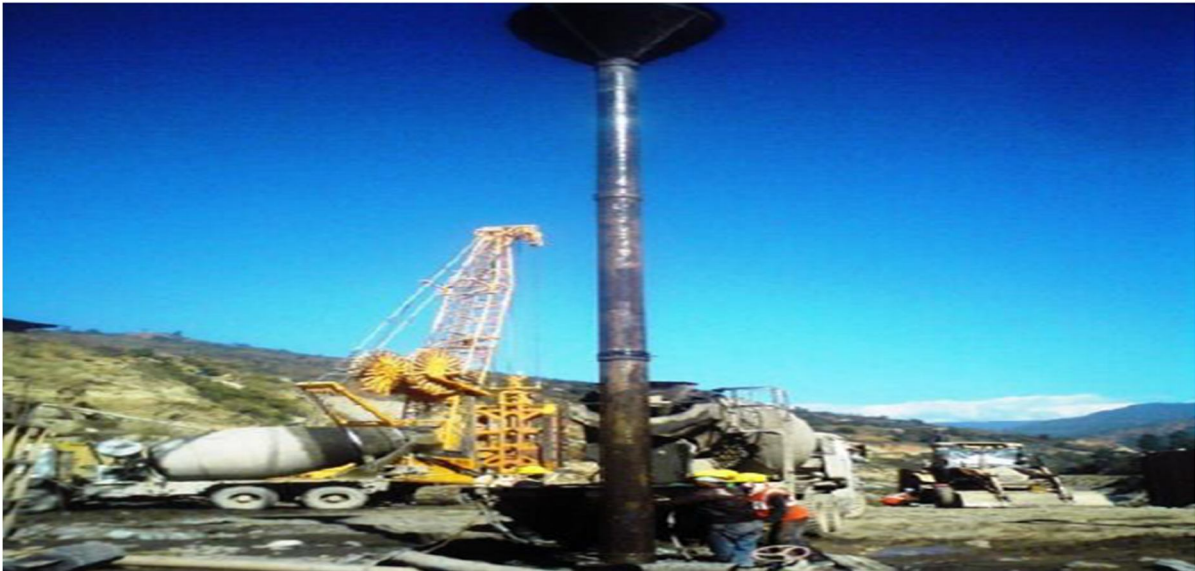
Fig 11.1. Concreting of Panels via Tremie
