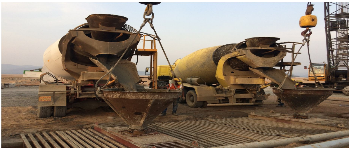
Fig 11.2. Concreting of Panels via Tremie
