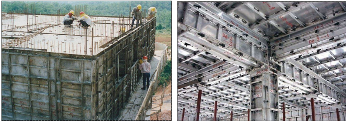
Figure 1.2 Mivan Formwork External and Internal View
