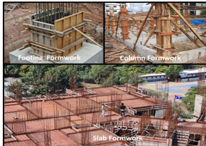
Figure 1.1 Conventional Formwork System
