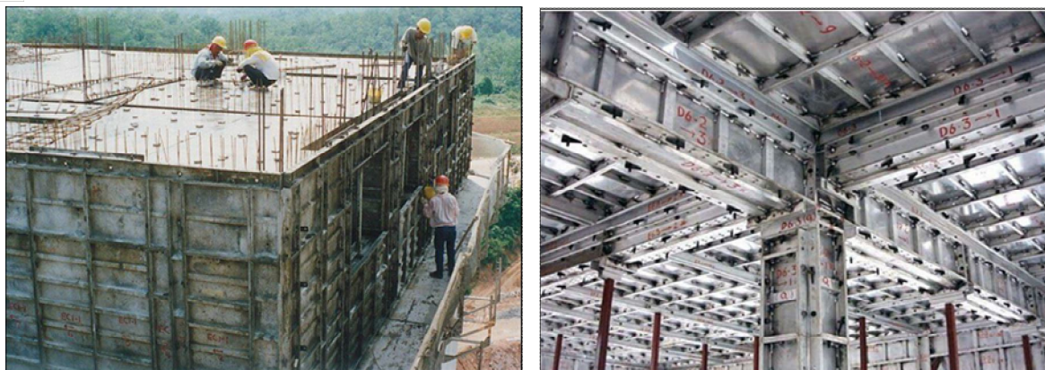
Figure 1.2 Mivan Formwork External and Internal View
