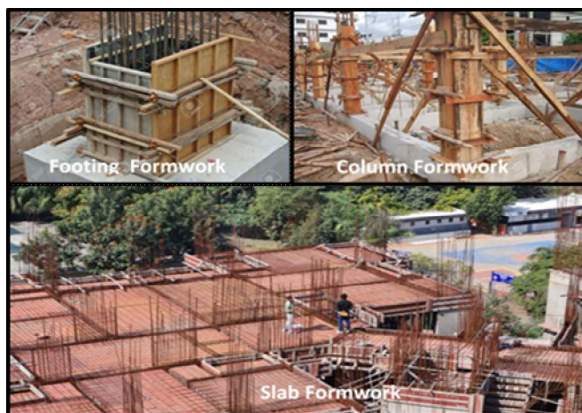
Figure 1.1 Conventional Formwork System
