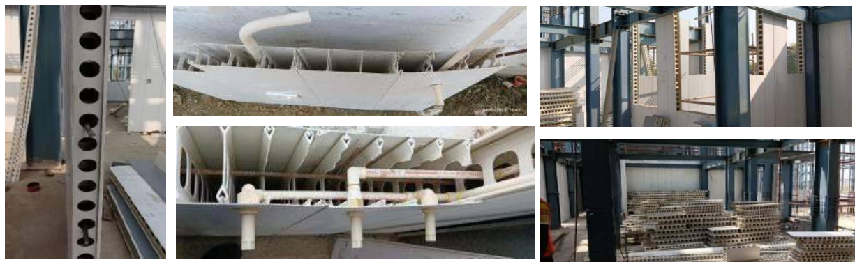
Figure 9: Wall Erection
