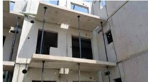
Figure 16: Precast cantilever balconies
