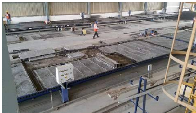
Figure 24: Steel casting beds for Precast slab
