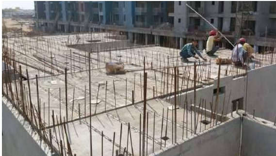
Figure 15: Precast half slab with lattice girder
