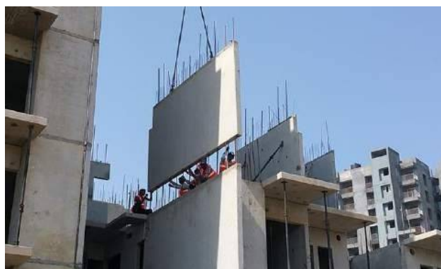
Figure 17: Erection of load bearing Precast wall panel
