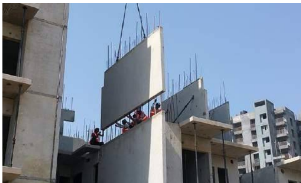
Figure 17: Erection of load bearing Precast wall panel
