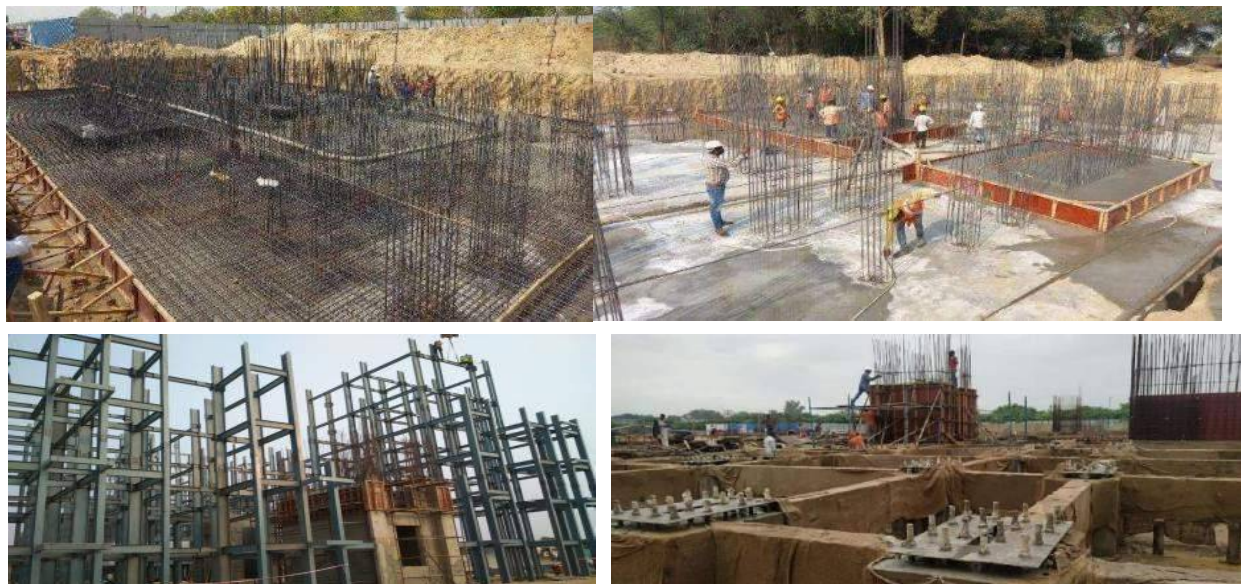
Figure 7: Foundation & Columns in L.H.P.
