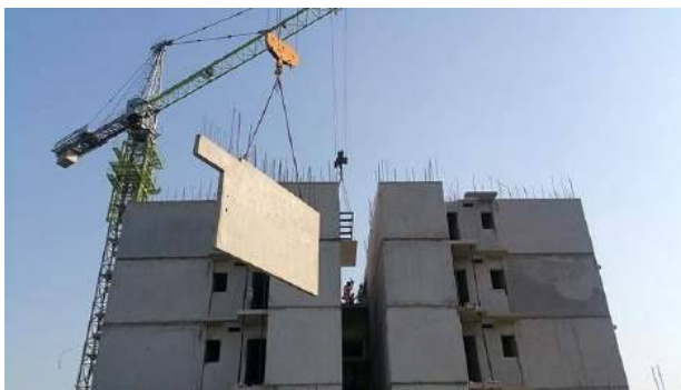
Figure 13: Precast concrete wall erection
