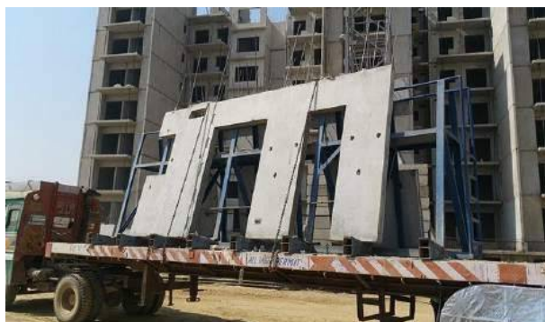
Figure 26: Transport of precast wall panels
