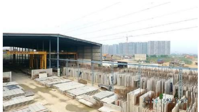
Figure 25: Stockyard for precast elements
