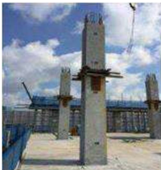
Figure3: Typical Precast Column Details
