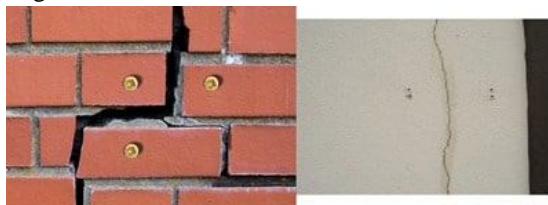
Fig.7: Installing three screws at right angle triangle to measure both shear and normal movement
