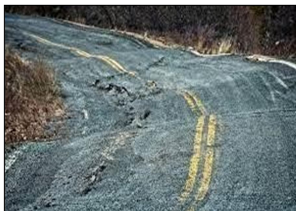
Fig 3.3: Crumbling infrastructure due to thawing of permafrost
