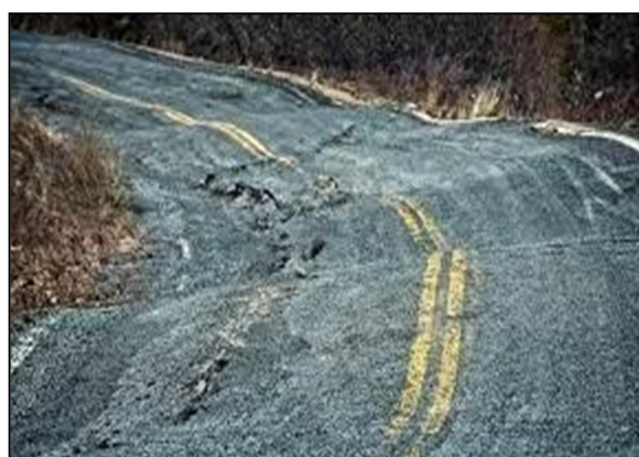
Fig 3.3: Crumbling infrastructure due to thawing of permafrost
