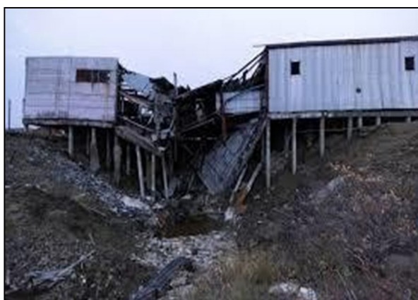
Fig 3.3: Crumbling infrastructure due to thawing of permafrost
