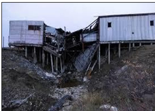
Fig 3.3: Crumbling infrastructure due to thawing of permafrost
