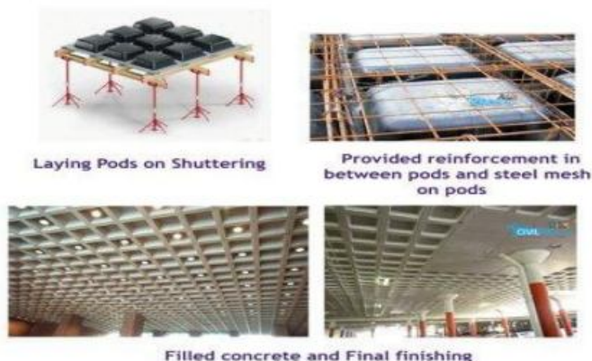
Figure 3: Waffle slab
