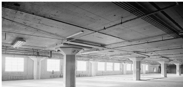
Figure 1: Flat slab
