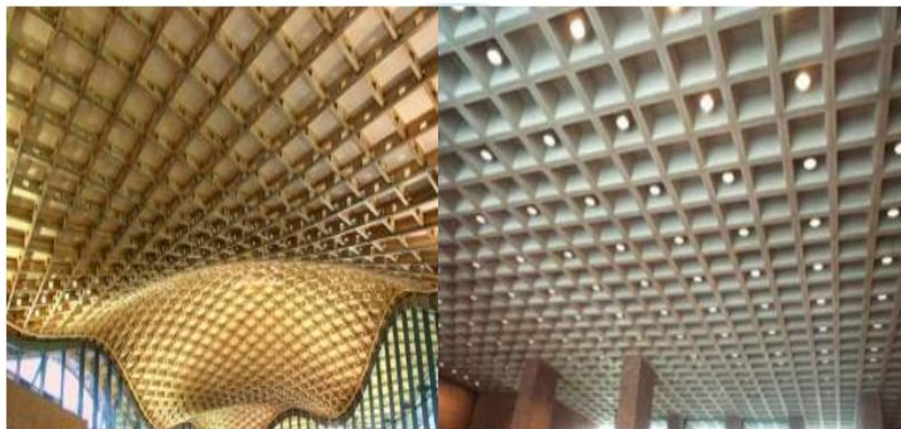
Figure 4: Grid slab
