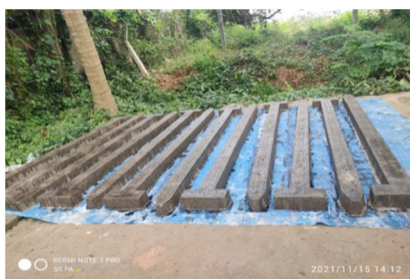
(Fig:- (4)- FINSHING OF FENCING POLE)
