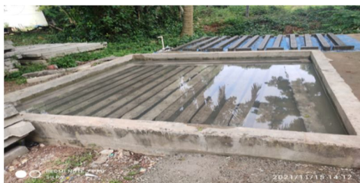
(Fig :- (3)-CASTING & CURING)
