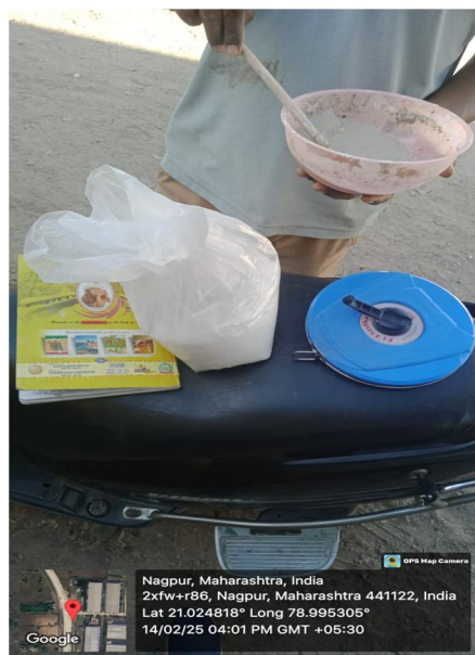
Fig. 4. Make a wet lime and necessary material
