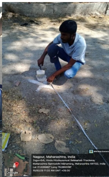
Fig. 5. After Mark the point use of wet lime
