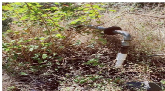
FIG 5. Existing Bore well
