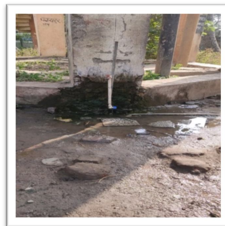
Fig. 3 Condition of existing ESR
