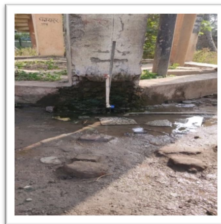
Fig. 3 Condition of existing ESR
