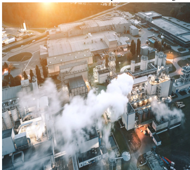
Fig.1. Industrial Waste Heat
