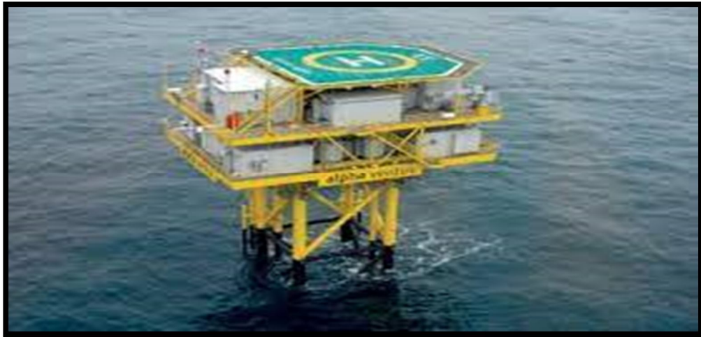
Fig.1 Shows Step-up Transformer
